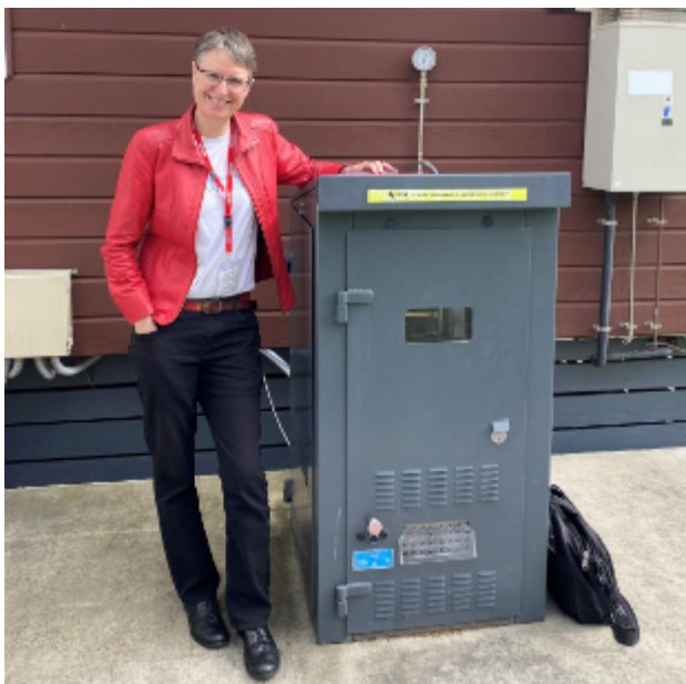
Sally Brooker with the Hylink household-sized robust electrolyser which produces green hydrogen from water and is powered by sun and wind. It was developed by Robert Holt and his team at Callaghan Innovation and provides instant hot water for showers, taps and radiators as well as fuel for the BBQ (Photo: Robert Holt).
